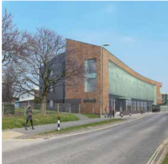
£9m upgrade to facilities at Eastleigh College
