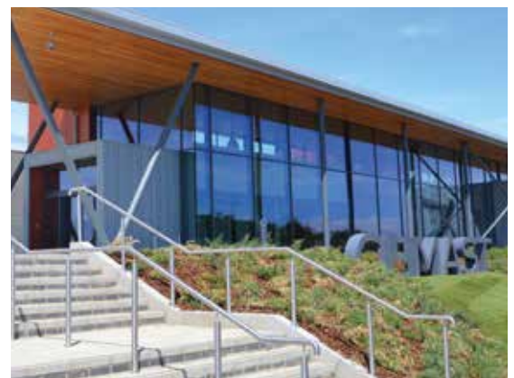
£12m CEMAST Centre at the Solent Enterprise Zone
