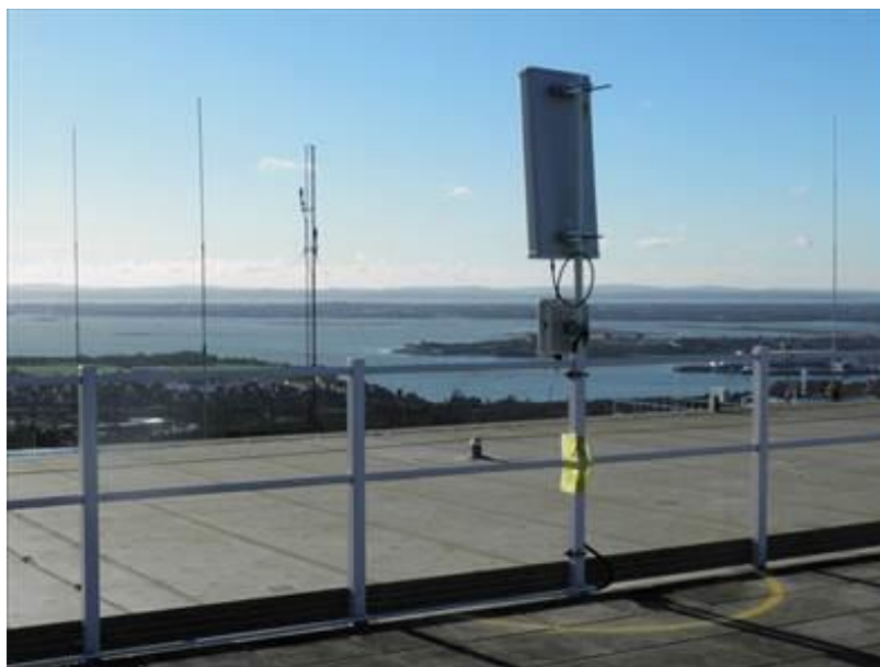
Figure 7: Example Radio Node at Portsdown Technology Park
