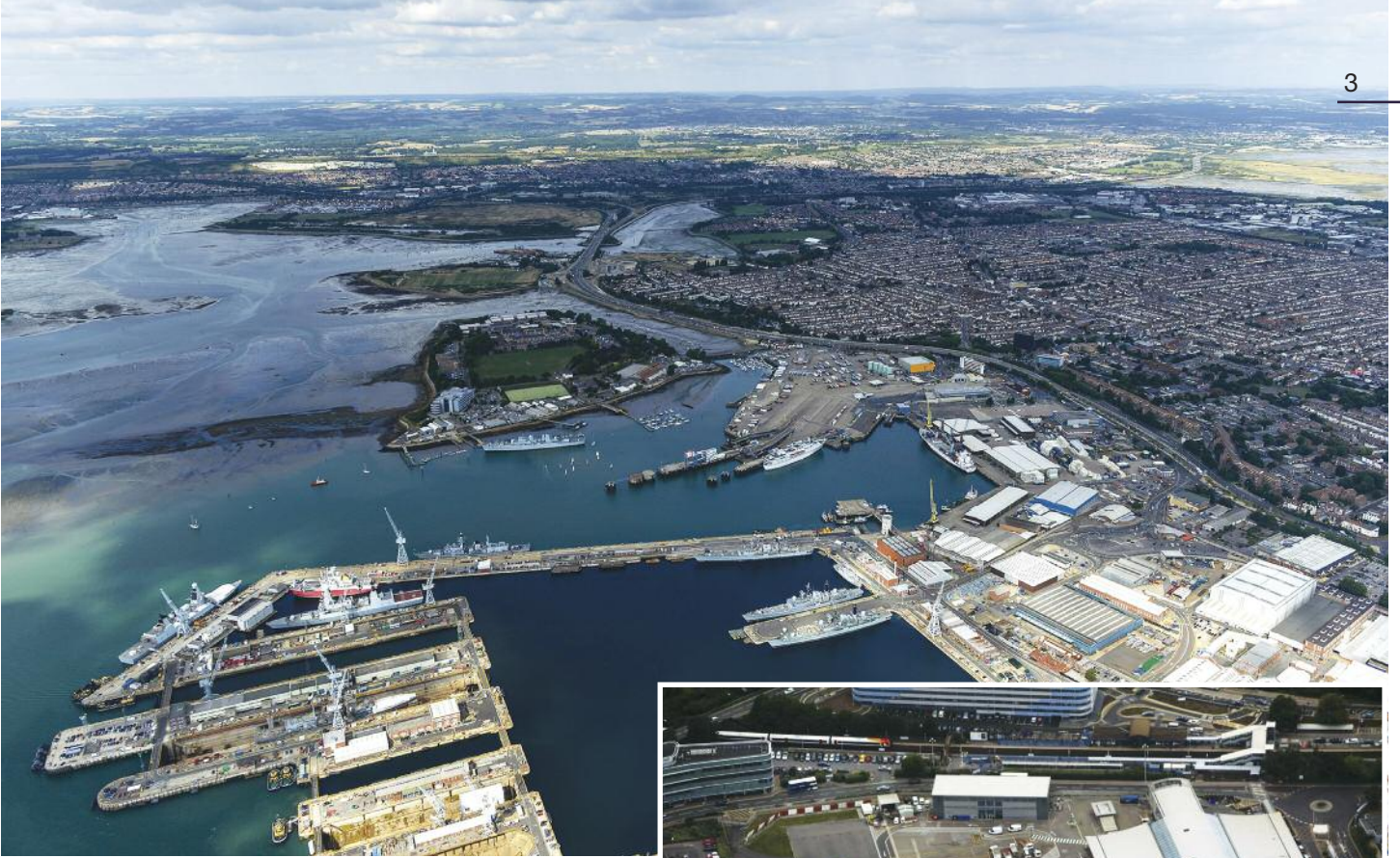
Centre of engineering excellence: Portsmouth Naval Dockyard
