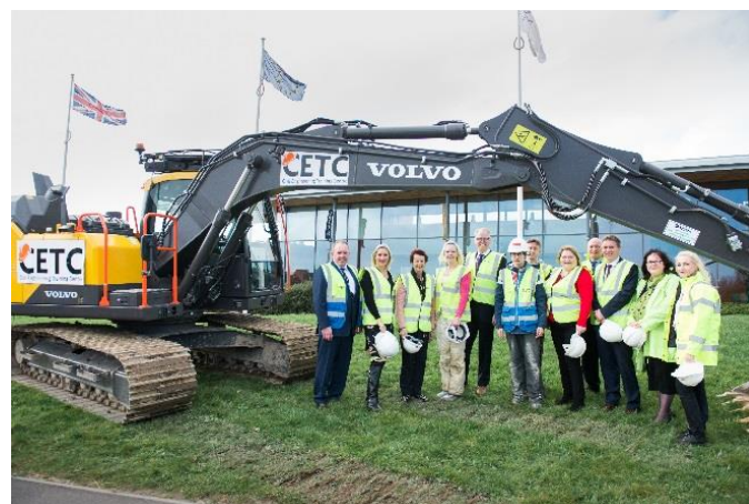
Construction works start at Fareham College's new £4.1m New Civil Engineering Training Centre
